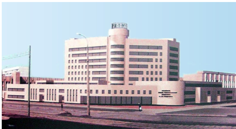
Figure 4 / H. 3 Building with the Russian-Swiss Education and Scientific Centre for pharmaceutical and biotechnologies transfer
