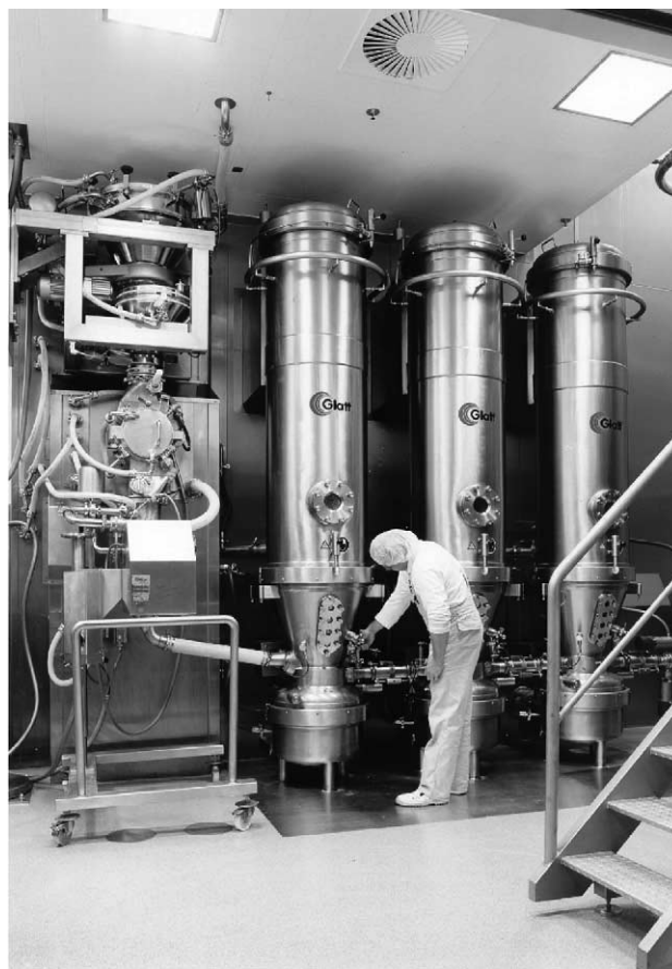
Fig. 5. Glatt Multicell® Production Plant at Pfizer Goedecke, Freiburg, Germany.
