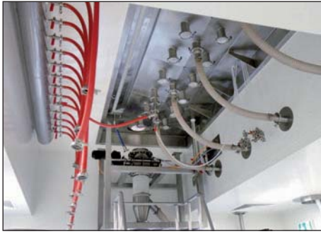
Level 0: Nozzle connections ProCell 250 (LH), spray tank and Big Bag filling station for product (RH)
