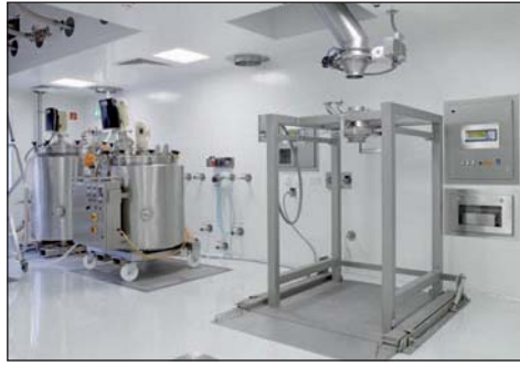
Level 0: Nozzle connections ProCell 250 (LH), spray tank and Big Bag filling station for product (RH)
